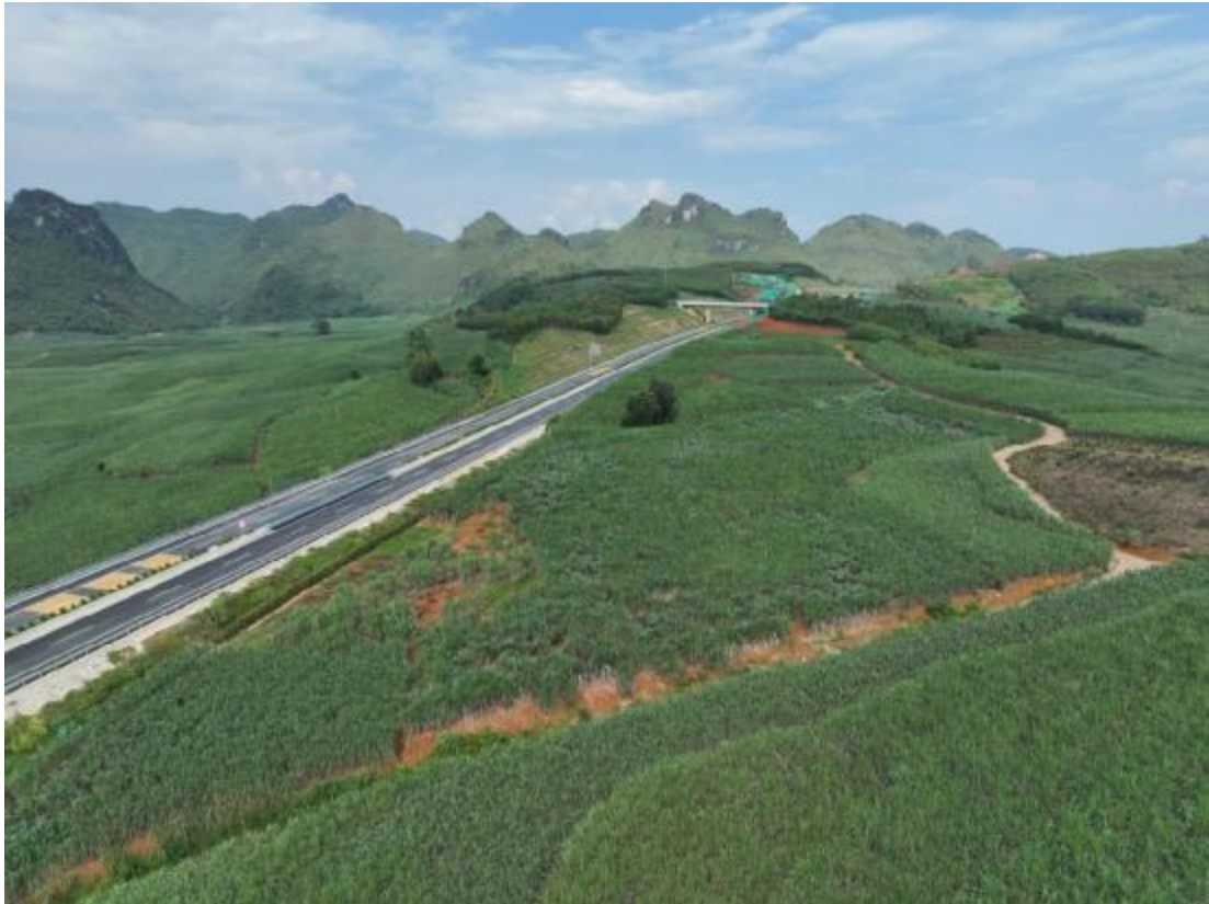
场地修整，撒播草籽，现复耕
